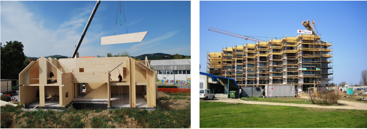
Fig. 2: Hose Crnile (left), Terme Catez upgrade (right)
